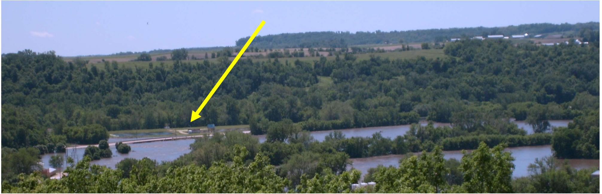
The wastewater treatment facility after the 2008 flood.
