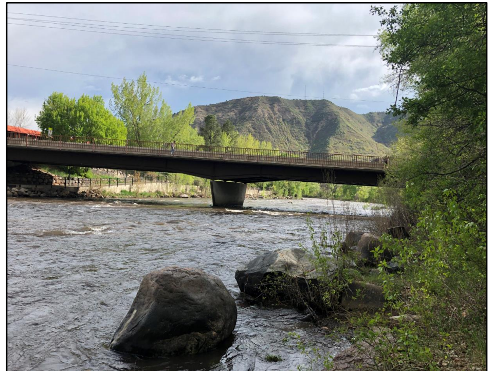
Photograph 8. Runoff flow conditions, Spring 2019
