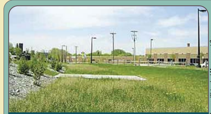
Biofiltration swale planted with native sweetgrass
