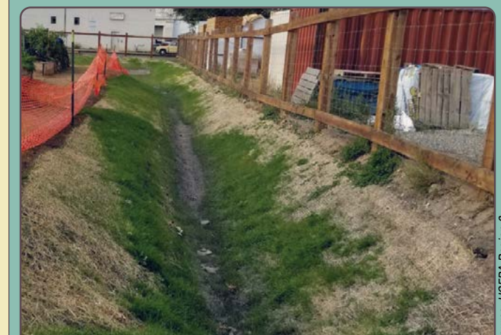
After: Within 6-12 hours the retained water has drained or infiltrated leaving a dry bottom
