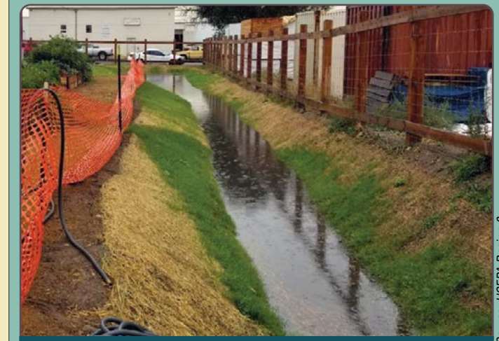
Before: This recently constructed biofiltration swale in a park in Helena exhibits shallow ponding of water after a rain event
