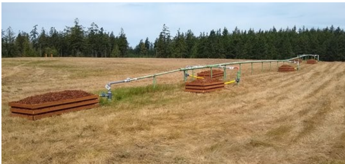
Biofilters at Jefferson County Landfill, Washington. Used with permission from Jefferson County and Aspect Consulting.
