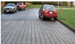
**Continuous Permeable Pavement** systems are excavated areas filled with gravel and paved over with a porous concrete or asphalt mix. **Block Paver** systems consist of impervious paver blocks placed on a sand or pea gravel bed with a gravel storage layer below.
