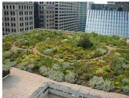
**Green Roofs** are another variation of a bio-retention cell that have a soil layer laying atop a special drainage mat material that conveys excess percolated rainfall off of the roof.
