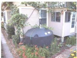
**Rain Barrels (or Cisterns)** are containers that collect roof runoff during storm events and can either release or re-use the rainwater during dry periods.
