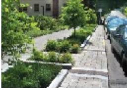
**Bio-retention Cells** are depressions that contain vegetation grown in an engineered soil mixture placed above a gravel drainage bed. They provide storage, infiltration and evaporation of both direct rainfall and runoff captured from surrounding areas.
