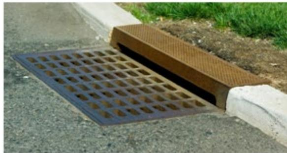
**Figure 3-3 Storm drain inlet**
