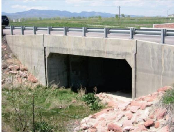
**Figure 3-2 Concrete box culvert**
