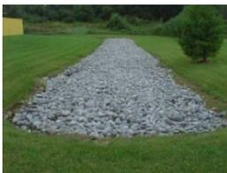
**Infiltration Trenches** are narrow ditches filled with gravel that intercept runoff from upslope impervious areas. They provide storage volume and additional time for captured runoff to infiltrate the native soil below.
