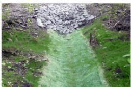
**Vegetative Swales** are channels or depressed areas with sloping sides covered with grass and other vegetation. They slow down the conveyance of collected runoff and allow it more time to infiltrate the native soil beneath it.
