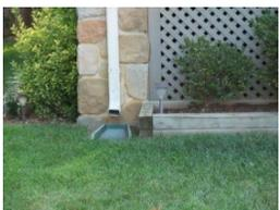
**Rooftop Disconnection** has downspouts discharge to pervious landscaped areas and lawns instead of directly into storm drains. It can also model roofs with directly connected drains that overflow onto pervious areas.
