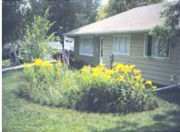
**Rain Gardens** are a type of bio-retention cell consisting of just the engineered soil layer with no gravel bed below it.
