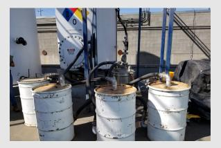
Cleanup using soil vapor extraction involves drilling one or more extraction wells into contaminated soil, and using a vacuum to pull air and vapors through the soil and up to the surface for treatment.
