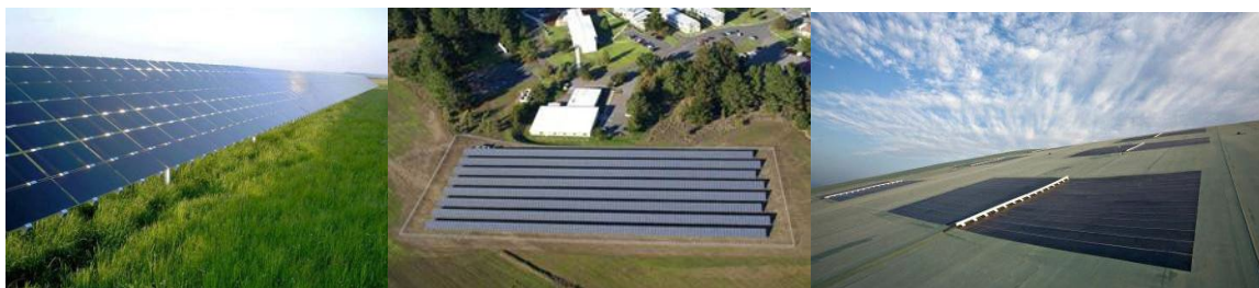
Figure 3-4: Thin-film solar modules installed on (i) solar energy cover and (ii/iii) fixed tilt mounting systems
