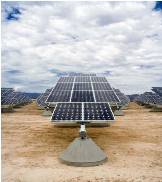
Figure 3-7: PV system with single-axis trackers installed on former landfill at Nellis Air Force Base, Nevada.
