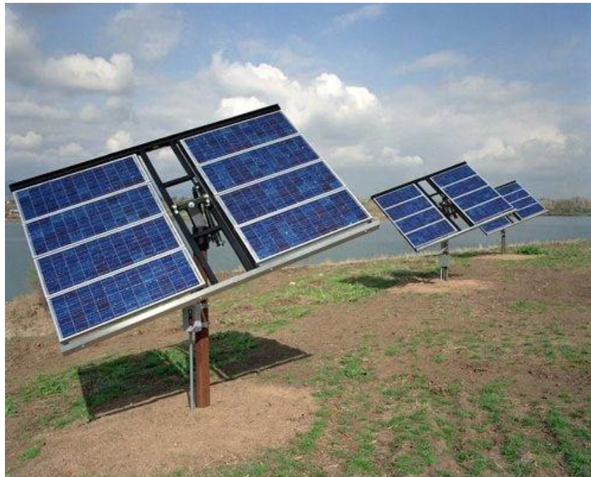
Figure 3-7: PV system with single-axis trackers installed on former landfill at Nellis Air Force Base, Nevada.
