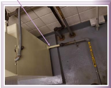
Figure 2: 50-gallons day tank with no shutoff valve and bottom connection incorrectly below the liquid level of the tank.
