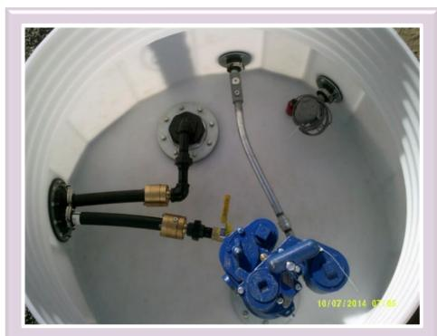
Figure 14: Sump containing submersible pump head, pressurized supply piping and a return pipe.
