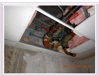
*Figure 8:* Illustration of aboveground piping in a ceiling (here ceiling tile moved to expose piping) that is exempt from federal UST technical prevention requirements.
