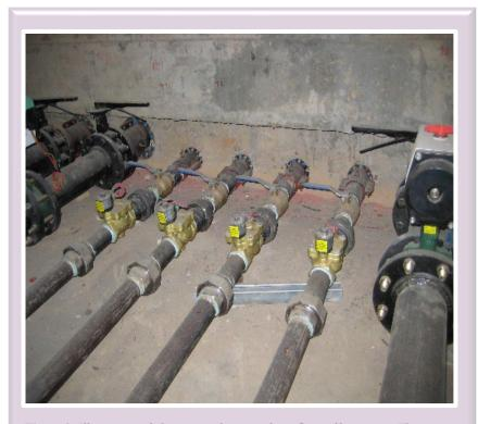
Figure 9: Illustration of aboveground piping above floor of basement. This section of piping is exempt from federal UST technical prevention requirements but may be subject to the SPCC regulation. Note that the section of the piping back to the underground tank (not shown) that is routed through the concrete, but most importantly is in contact with soil, must meet federal UST release detection requirements.
