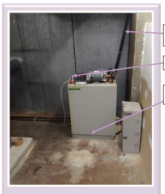
Figure 1: 50-gallons single-wall day tank with improper supply and return lines, no emergency venting, and no secondary containment.
