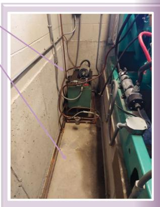
Figure 4: 10-gallon day tank with improper material for vent line and insufficient room for inspection and repair.
