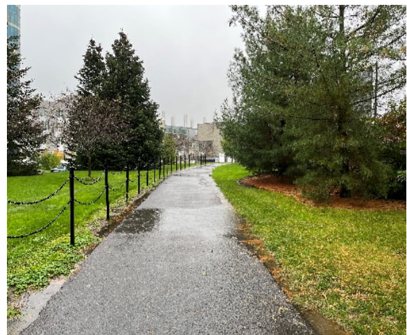
Figure 5. Pooling on walkways near Hoy Field.
