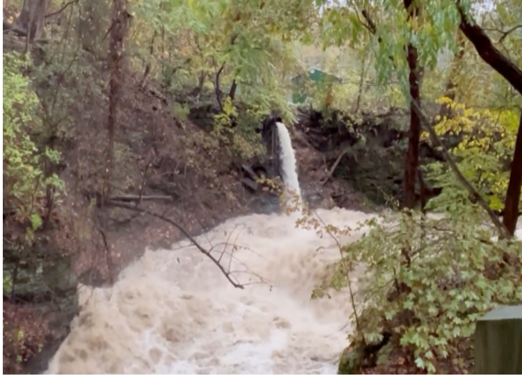
Figure 6. Stormwater discharge into Cascadilla Gorge in the south portion of our site.
