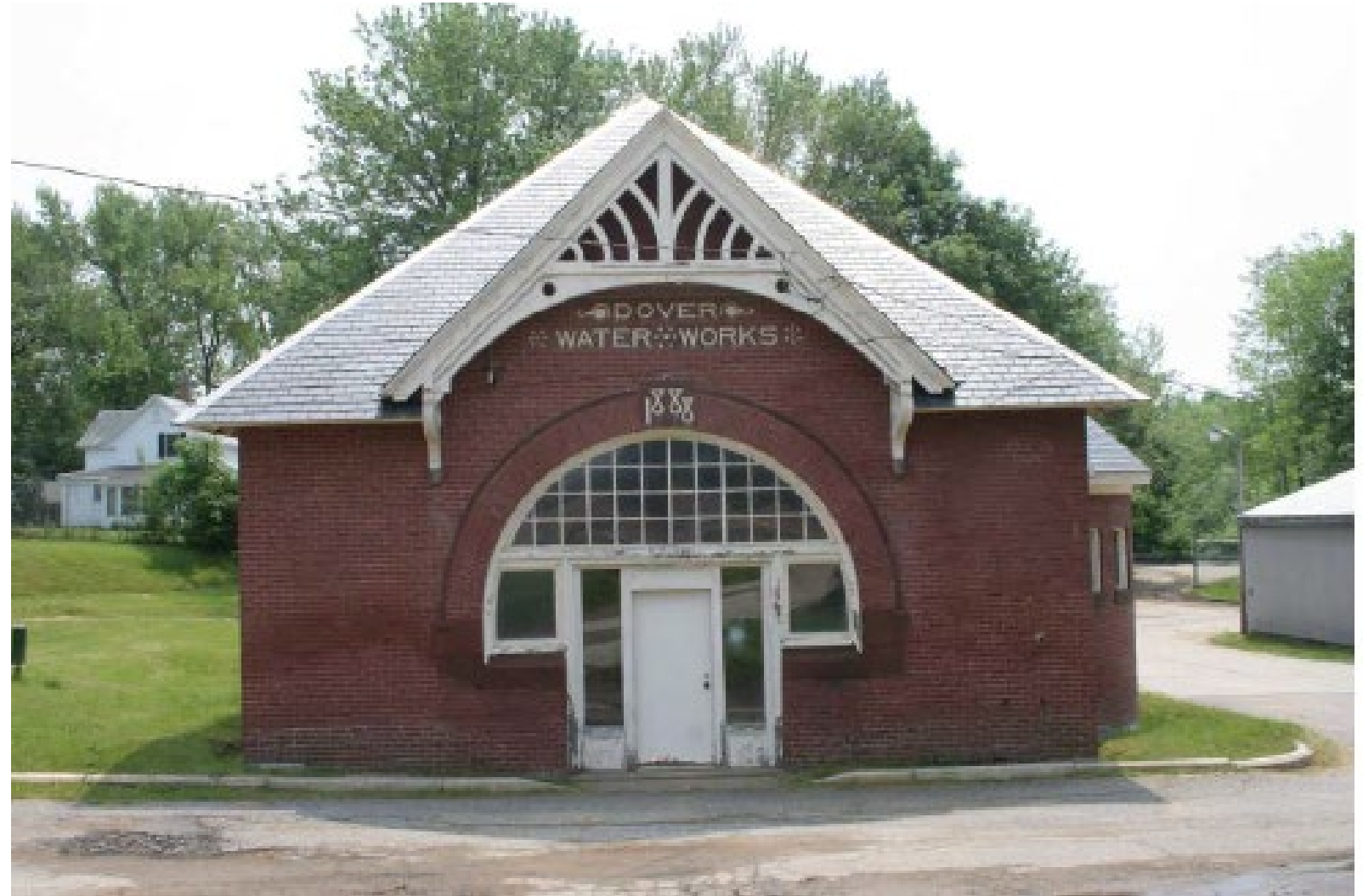
Historic Municipal Water Works, Dover, NH
