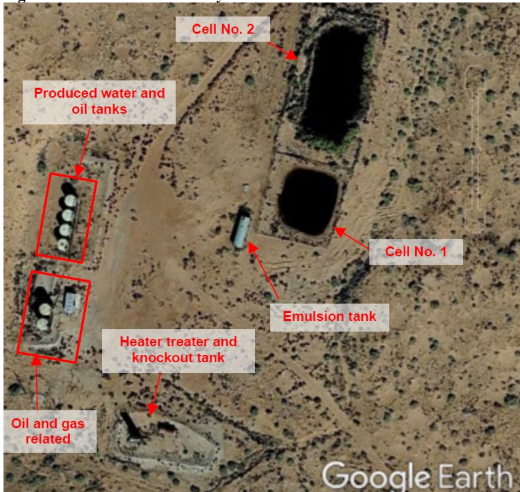
Figure 4: Aerial view of Battery No. 3
