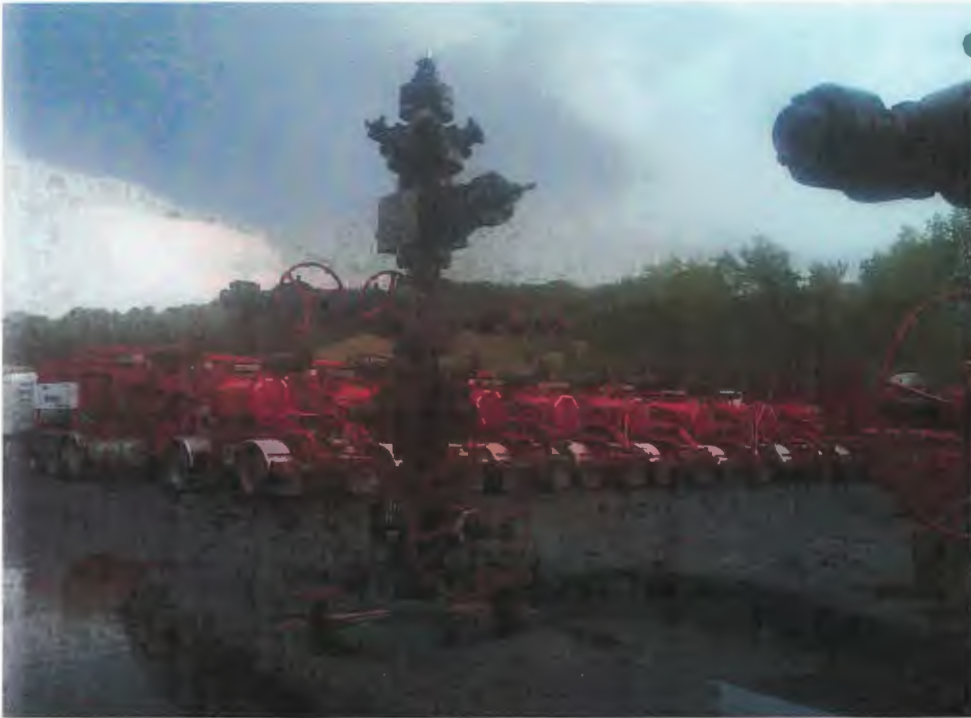
Unconventional Well Completion Fleet (hydrofracture)
