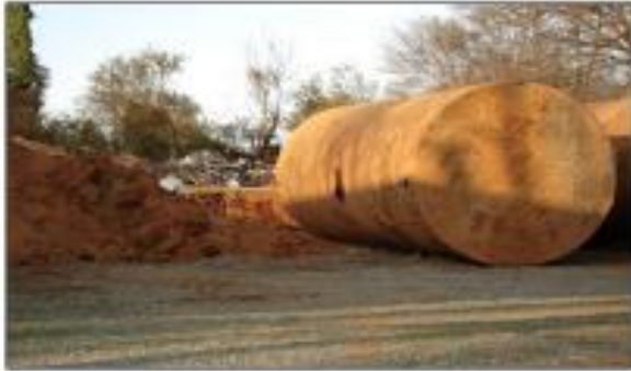
Removal of 20,000 gallon Underground Storage Tanks Leaking Cancer Causing Petroleum (1/15/08)
