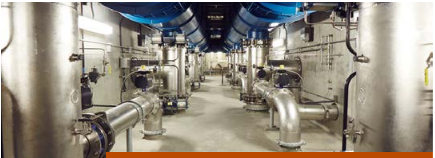
Photo Courtesy of Orange County Water District
