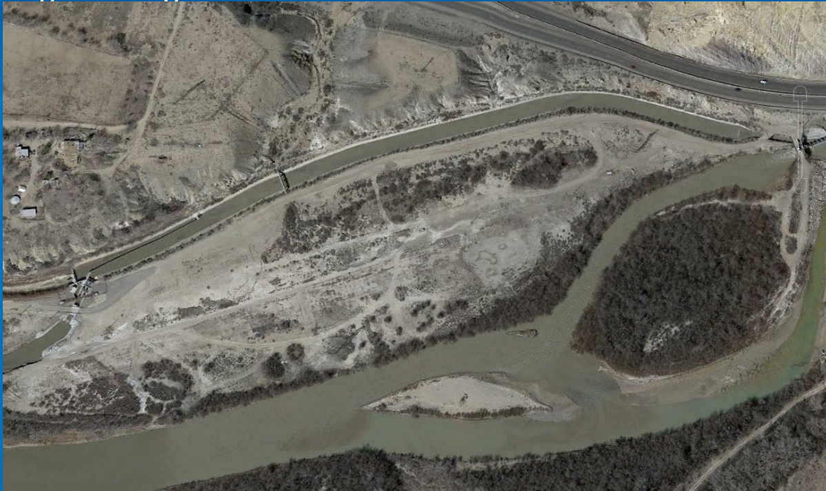
Hogback irrigation canal
