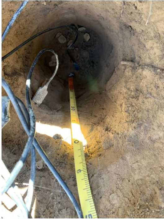
Soil moisture & temperature
