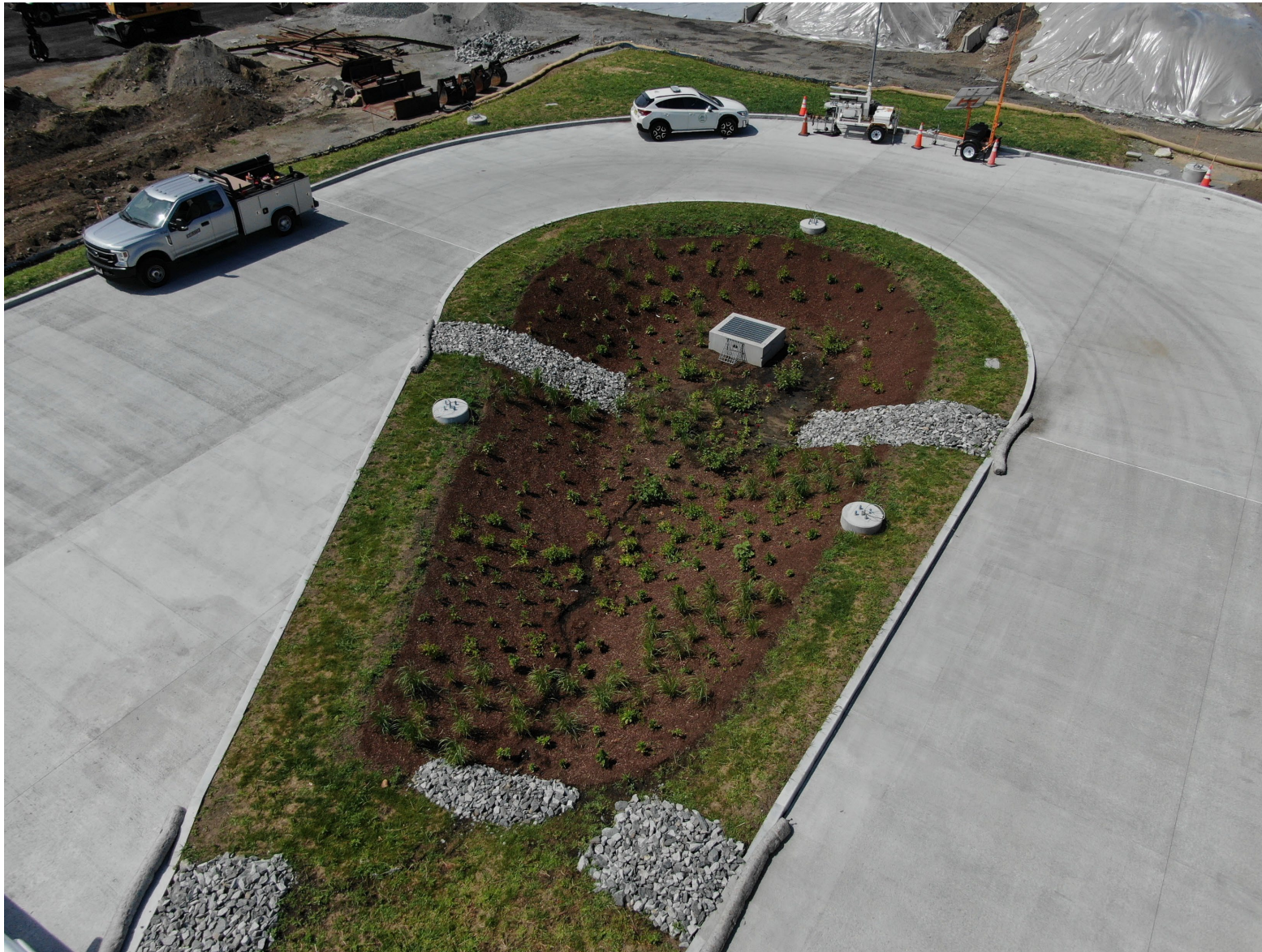
Source: Rhode Island Department of Transportation Bio-Filtration Basin at Pawtucket/Central Falls Transit Center
