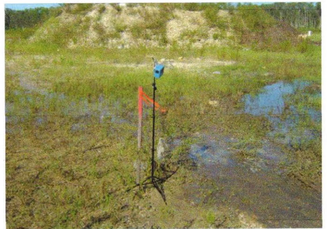
④ Photo 4. Area air monitoring during soil removal.
