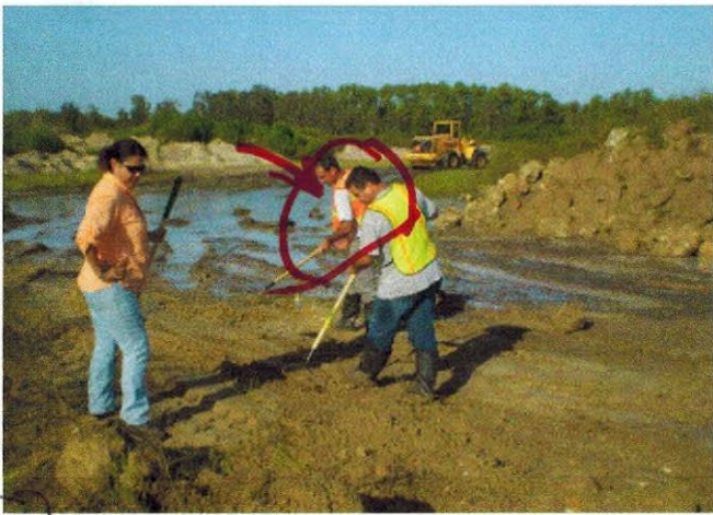
Photo 7. Workers utilizing hand tools to survey soil for asbestos fragments.
