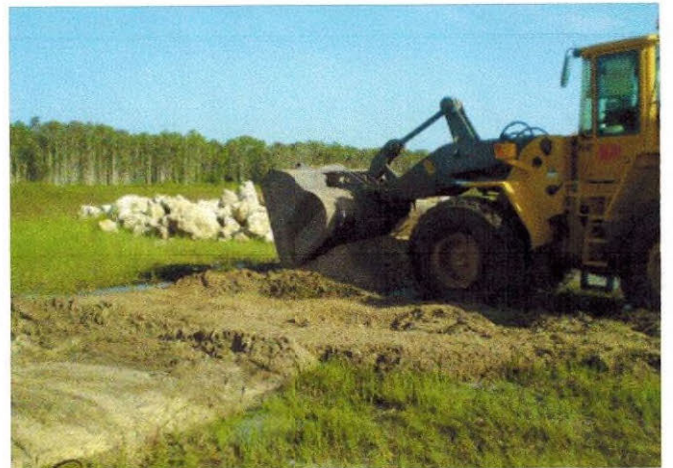
⑥ Photo 6. Loader spreading soil to be surveyed for asbestos fragments.
