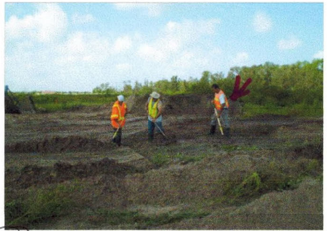
Photo 8. Workers surveying soil for asbestos fragments.
