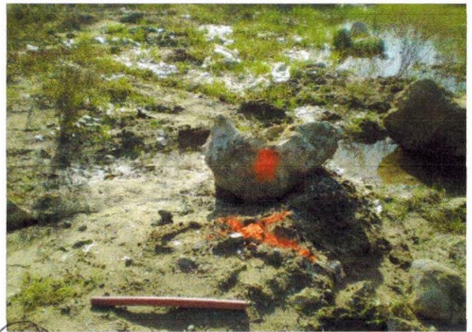
Photo 10. Asbestos fragments identified and removed.
