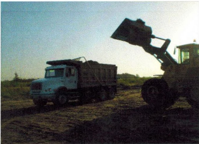
Photo 11. Contaminated soil disposed of in transport truck.
