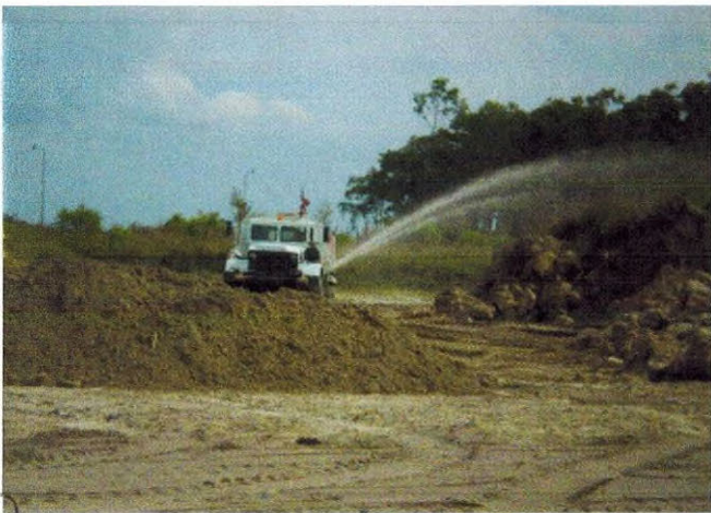
Photo 9. Water truck utilized to keep soil wet during removal.
