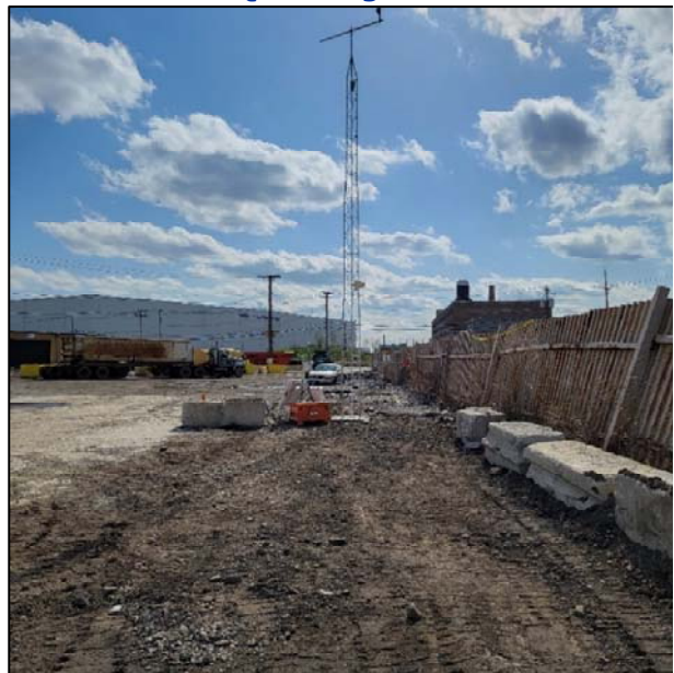
AQ1 Facing West
