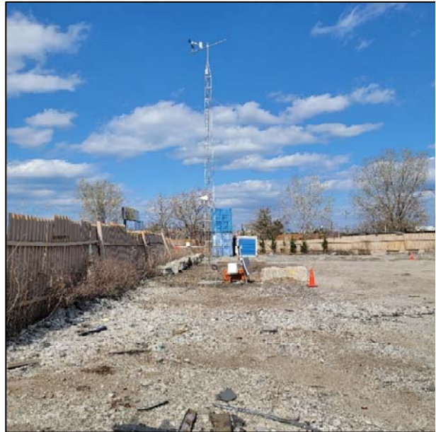
AQ1 Facing East
