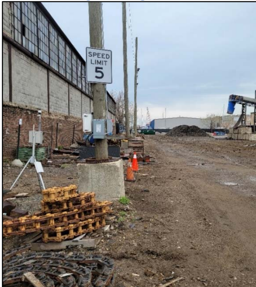
AQ2 Facing South
