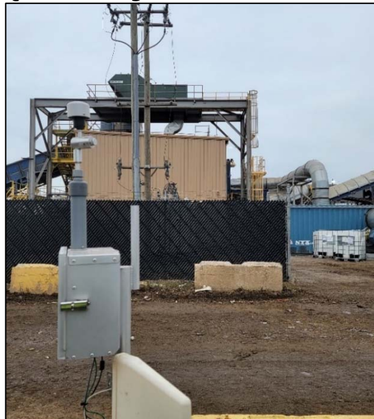
AQ3 Facing East
