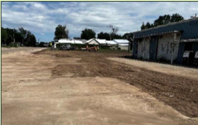
Land ready for a new business after underground tank removal.
