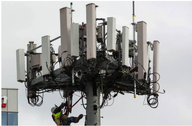
Technician repairs cell phone tower. Photo: Loren Holmes/Alaska Dispatch News/Zuma Press
