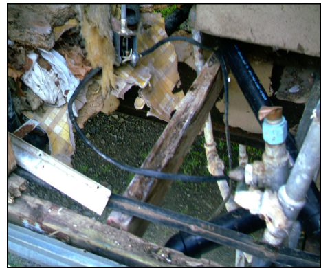
Photograph depicting the rotted floors of MHU2. The floor cavities were exposed raising a safety concern
