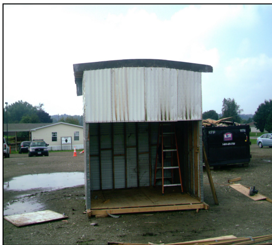
The main reconstruction project, the tool shed; 12 feet high by 6 feet wide.
