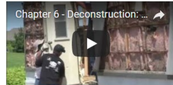
Chapter 6 - Deconstruction: Unit 1
