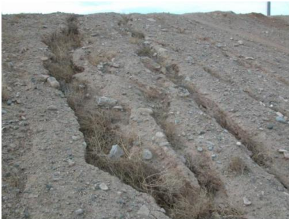
Figure A-1. Gully Formation Measured Over Six-Feet Deep in Albuquerque, NM
