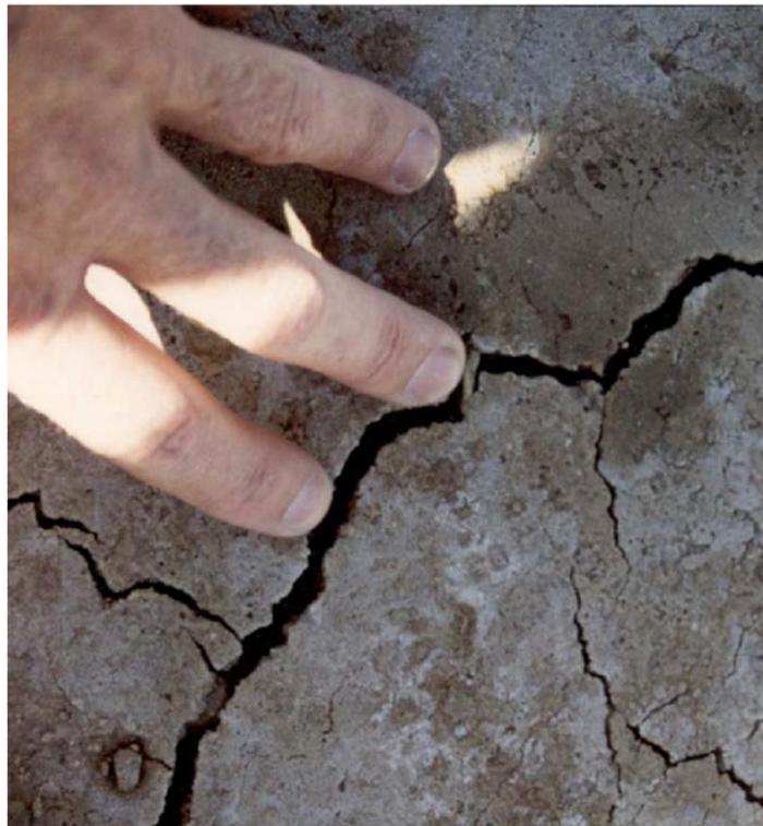
Figure 7. Desiccation Cracking in Clay Barrier Layer
