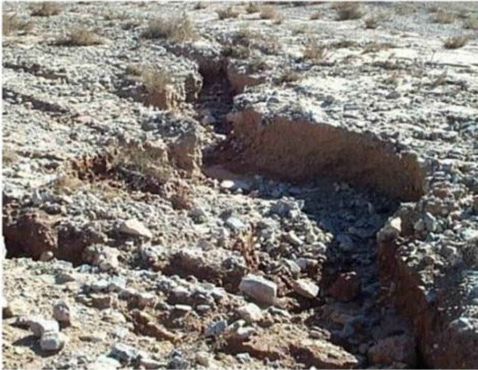
Figure B-1. Excessive Gully Erosion on Shallow Slope
