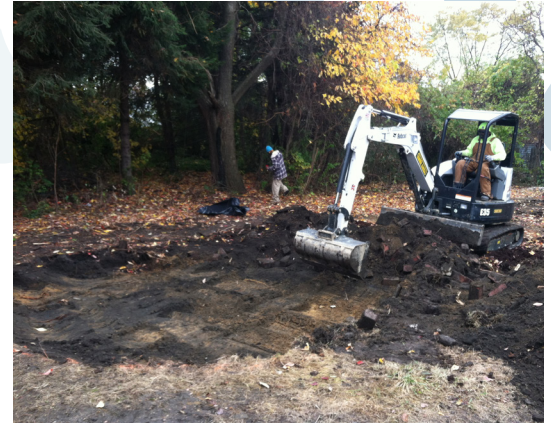
Excavation of vacant lot. Courtesy of the Cleveland Botanical Garden.
