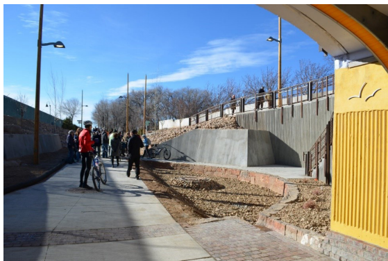
A semi-circular infiltration pond and the 15,000-gallon cistern prevents flooding and standing water on the trail when it rains. Courtesy Serquis + Associates and the City of Santa Fe
