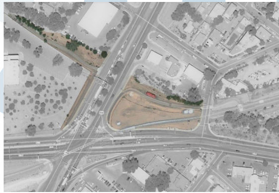
Arial image of St. Francis Drive Intersection before the project. Courtesy Serquis + Associates
