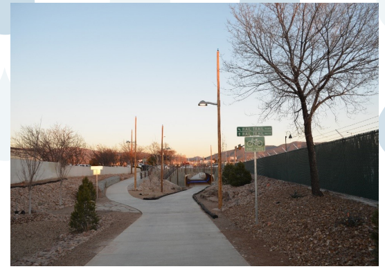
Finished trail and underpass. Courtesy Serquis + Associates
