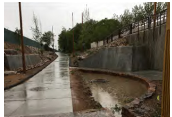
A semi-circular infiltration pond and the 15,000-gallon cistern prevents flooding and standing water on the trail when it rains. Courtesy Serquis + Associates and the City of Santa Fe
