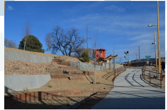
The underpass was excavated to resemble a canyon and the local landscape. Courtesy Serquis + Associates
