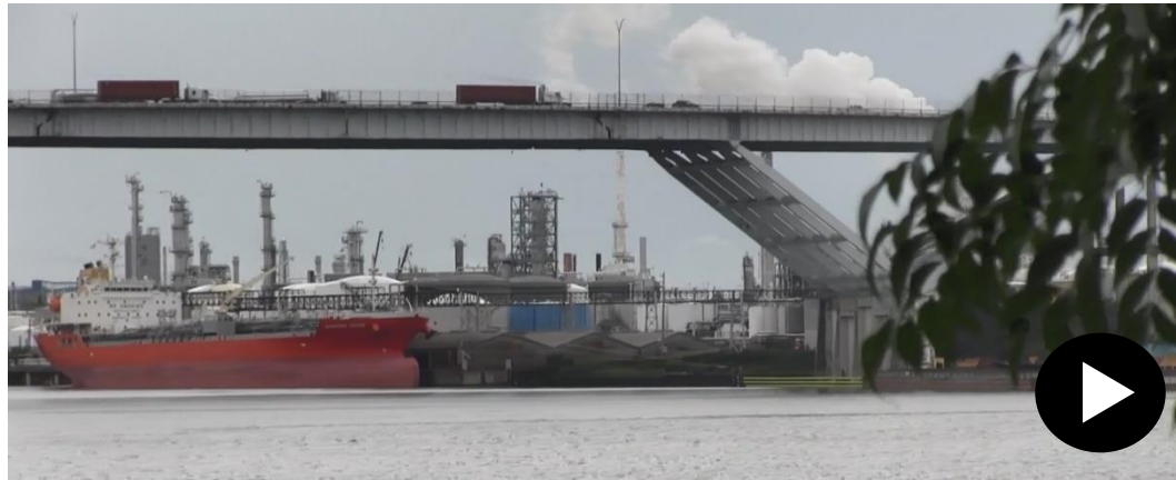
Ship Channel Bridge, Houston. (OIG video)
