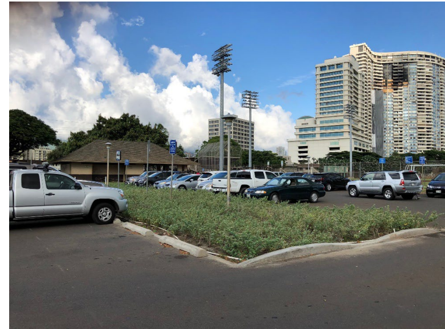
Bioretention Basin at Ala Wai Neighborhood Park
