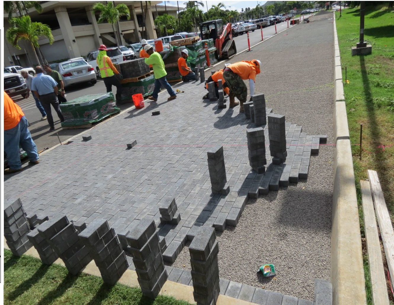
Permeable Pavement at Ala Wai Golf Course
