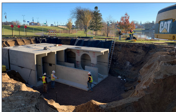
Figure 2. Installing the underground stormwater retention and filtration treatment facility in 2020.
