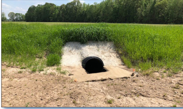
Figure 2. Grade stabilization structure BMP.
