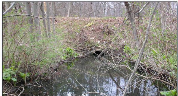
Figure 1. Culverts like this one on Eastman Avenue blocked fish passage and contributed to low DO.
