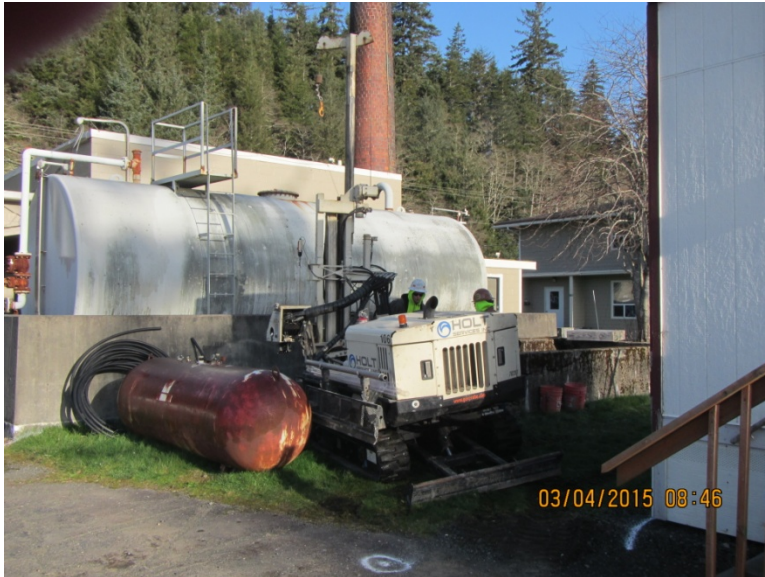
Photo 5. Drilling at USTs C/D (GP-11-CD3)
