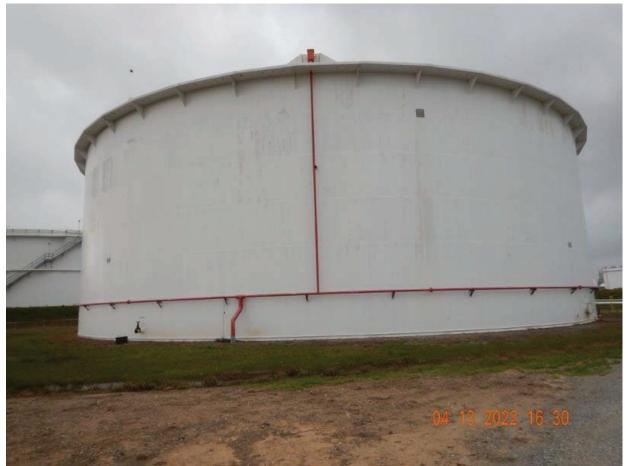
Photo File Name: DSCN0704.jpg Date of Photo: 4/13/2022 Time of Photo: 16:30 Photographer: Ben Rosenthal Description: Tank T-86. OGIC-visualized hydrocarbon emissions were observed on the roof of the tank.
