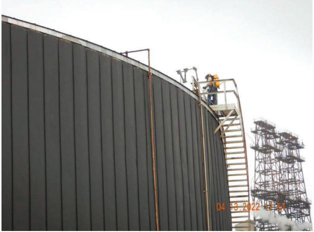
Photo File Name: DSC0708.JPG Date of Photo: 4/13/2022 Time of Photo: 17:51 Photographer: Ben Rosenthal Description: Facility LDAR technician using handheld monitoring equipment at the top of T-2001.
