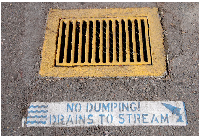
This storm drain stenciling design is easy to apply and provides a clear message to passersby that the drain leads to a stream.
