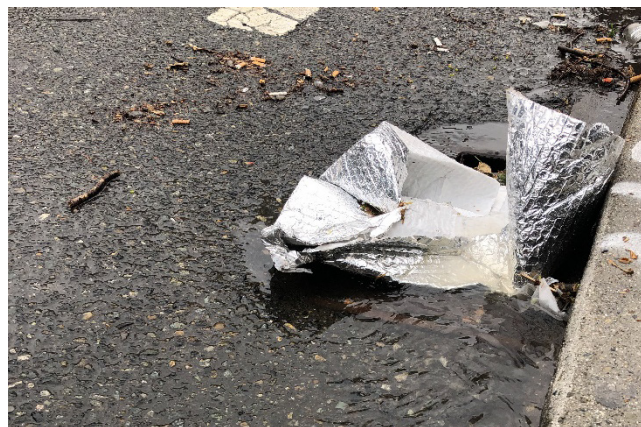
When not properly managed, trash can accumulate in storm drains where it can clog the systems and discharge into local waterways.
