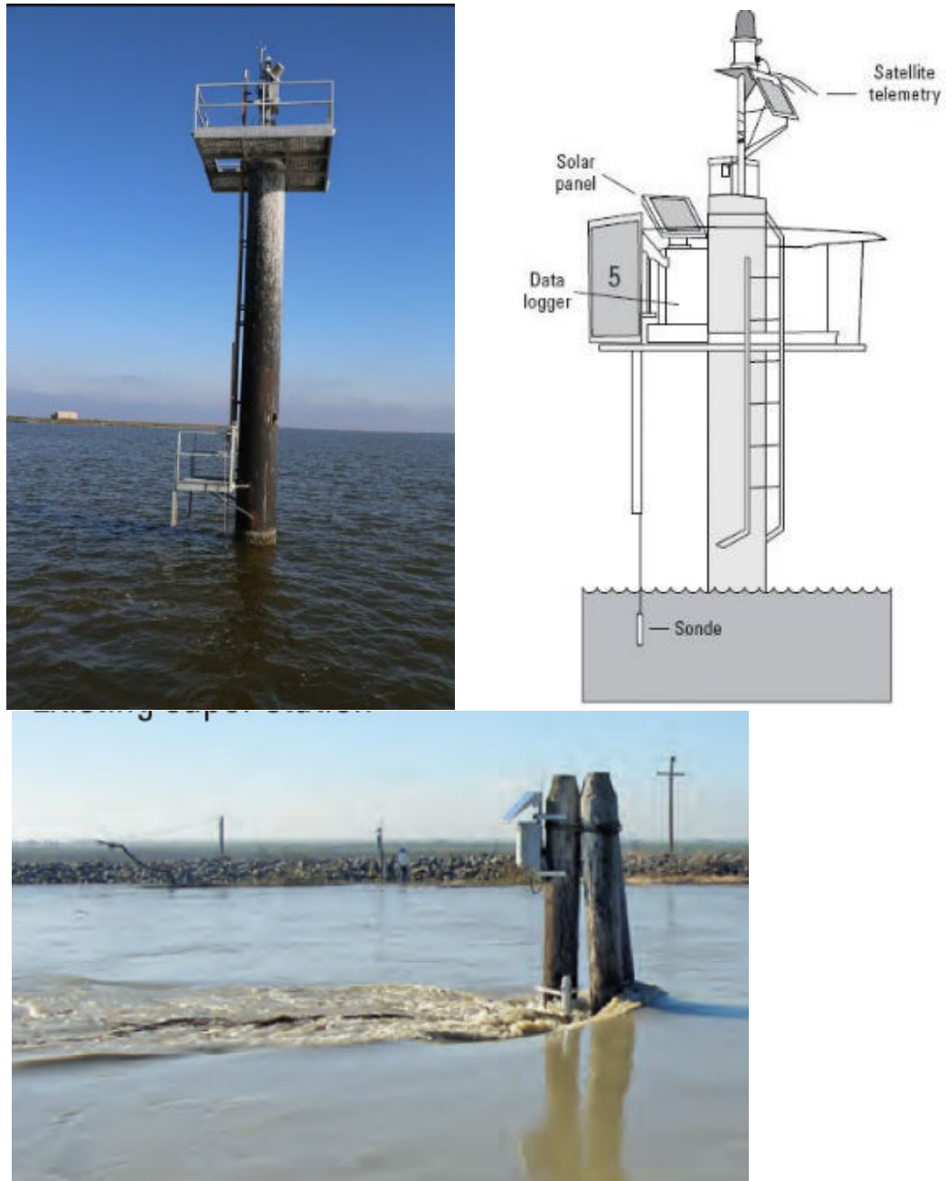
Figure C-1. Examples of Pier Mounted Monitoring Stations
