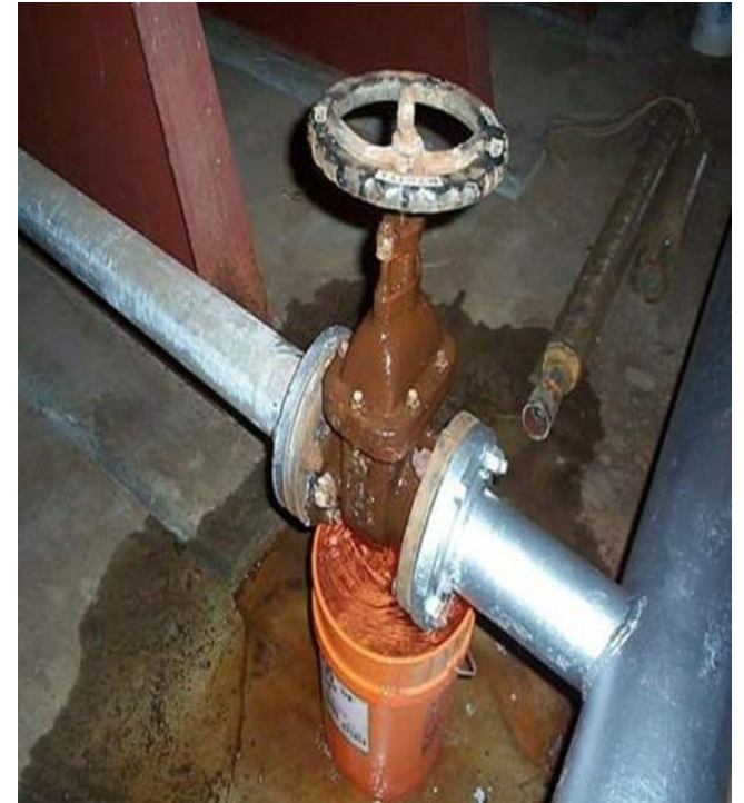
Leaking valve
