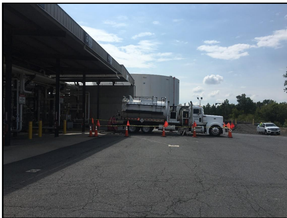
Picture 2: Vacuum Truck Extraction of Groundwater at Monitoring Well MW-34
