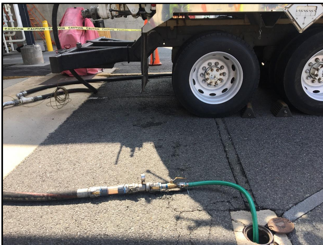
Picture 2: Vacuum Truck Extraction of Groundwater at Monitoring Well MW-34
