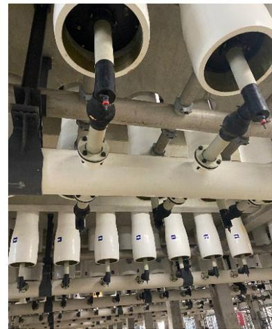
Vertical reverse osmosis technology is a space-efficient treatment option in use at the Sorek Desalination Plant.
