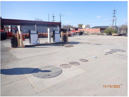
Description: Two 800 gallon fuel storage tanks are underground. One is for diesel and one is for
