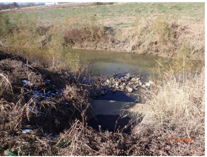
Description: Discharge of the Parkside Pump Station to Harding Ditch. The flapper gates to prevent water from Harding Ditch from backing up into the pump station still need to be repaired.
