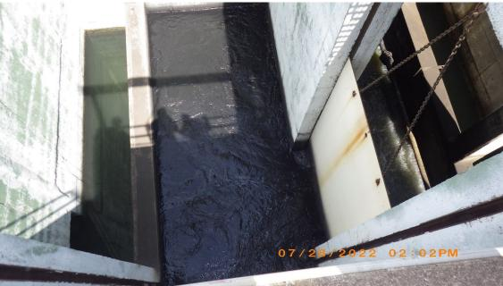
Description: Looking down into Manhole 120. There was an overflow event from this manhole to the Storm Ditch on 7/23/22 when power was disrupted to Wastewater Pump Station I. Location: Manhole 120.
