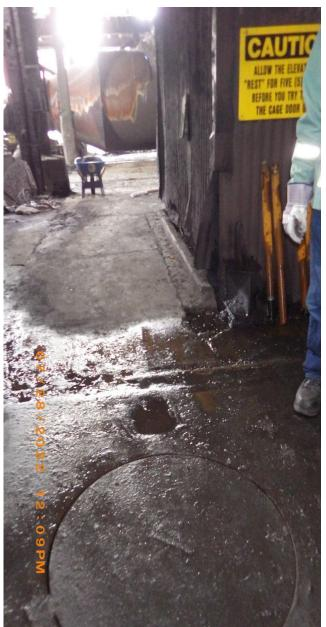
2: CHWW0058 Description: Manhole storm sewer cover under Blast Furnace C. During SWPPP inspection this cover was found removed. Location: Under Blast Furnace C. Date/Time: July 28, 2022/12:09 P.M.
