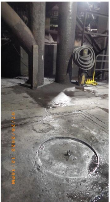
Description: Manhole storm sewer cover under Blast Furnace D. During SWPPP inspection this cover was found removed. Handle in the middle of the cover is a trip hazard and will be removed. Two large pipes in the background are pipes for non-contact cooling water. Location: Under Blast Furnace D. Date/Time: July 28, 2022/12:16 P.M.
