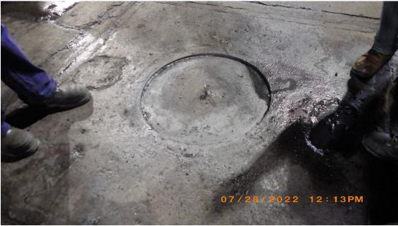
Description: Manhole storm sewer cover under Blast Furnace D. During SWPPP inspection this cover was found removed. Handle in the middle of the cover is a trip hazard and will be removed.
