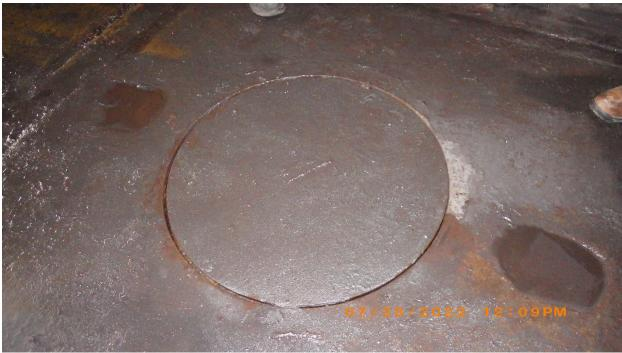
1: CHWW0057 Description: Manhole storm sewer cover under Blast Furnace C. During SWPPP inspection this cover was found removed. Location: Under Blast Furnace C. Date/Time: July 28, 2022/12:09 P.M.
