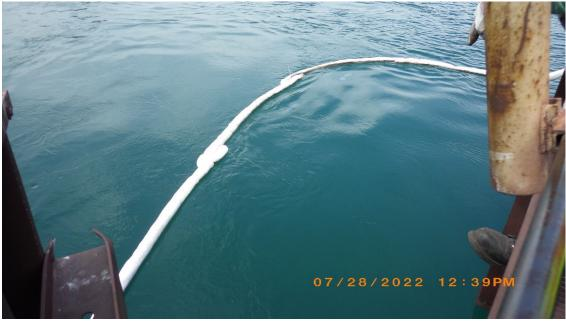
Description: Temporary, soft boom outside of Outfall 002 will catch any remaining foam that passes the permanent boom.
