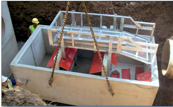
Figure 2. Installation of a baffle box at Infall 21.
