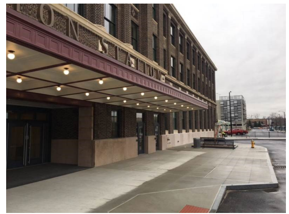
Figure 1: Front Entrance Credits: EPA
