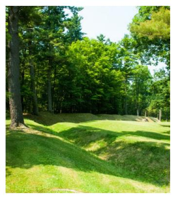
Figure 14. Grass Swale. (Source: USEPA 2021c)
