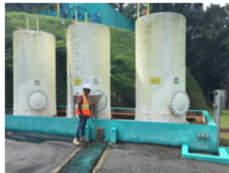
Earthquake Response: EPA facility assessment in Puerto Rico
