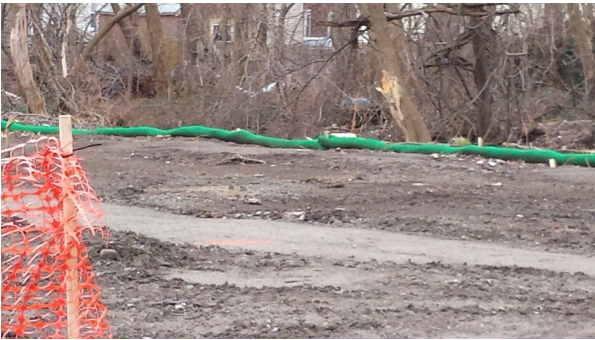
The Park under construction (photo credit: City of Brockton)
