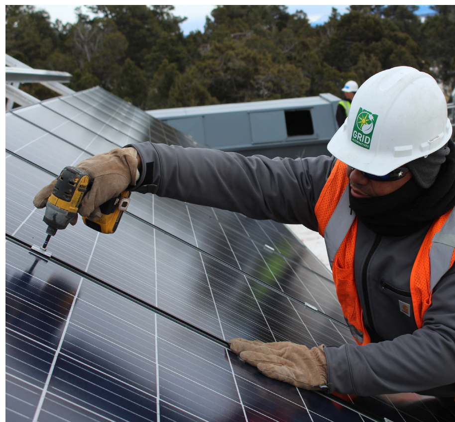
Installation of the San Miguel community solar array in Norwood, Colorado.
