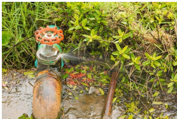
A leaking hose spigot
