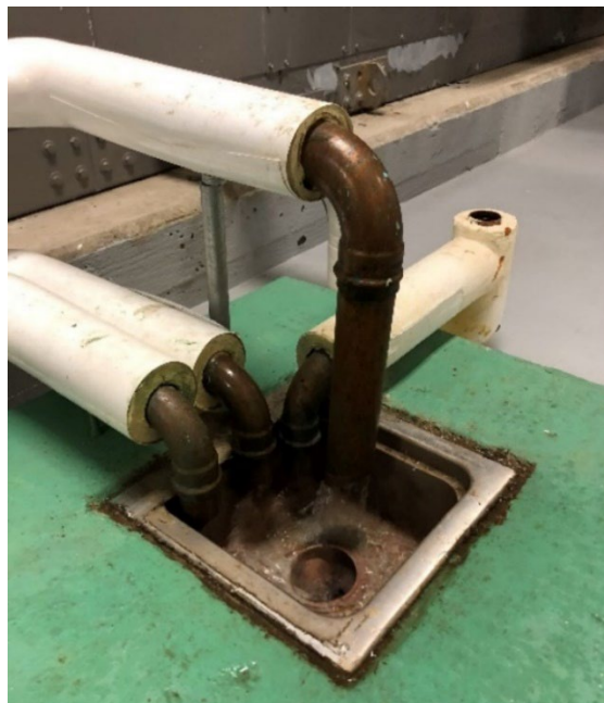
Condensate from an air handler flowing to a floor drain, which is a non-potable water source that could be used for cooling tower make-up water or other non-potable uses
