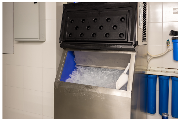
Ice maker lid left open when not in use, letting cool air out of machine
