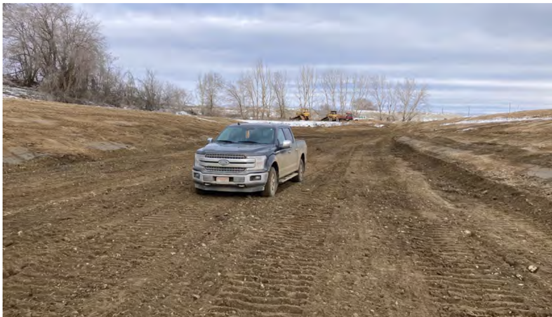
Photograph 1 Condition of Lagoon No. 3 in December 2021 Following Manure and Liquids Removal
